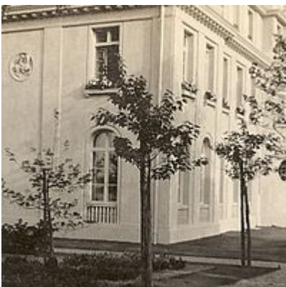
The north side of the villa
